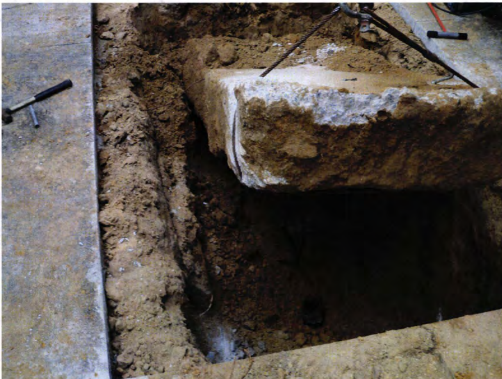
Picture 2: Concrete cap being lifted from UST 1192Bobwhite.
